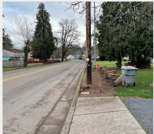
While sidewalks exist on the northern extent of 18th Ave, gaps remain to the south. South of the Boys and Girls club, there is a significant gap on the west side of the roadway. There are right of way constraints that prevent the continuation of the sidewalk.
