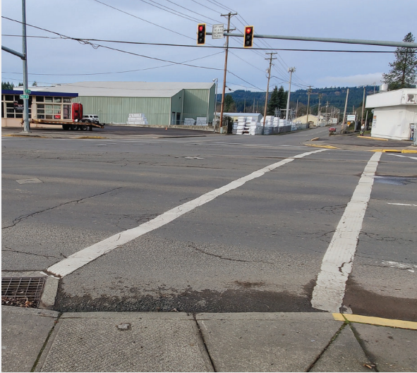
The intersection of Hwy 20 and 18th Ave is signalized, but long crossing distances and high traffic volumes make the intersection uncomfortable for pedestrians and bicyclists.
