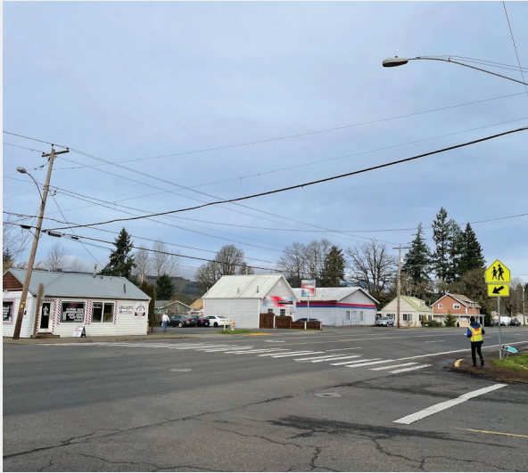
At the intersection of 22nd Ave and Hwy 20, there is a crosswalk that crosses five lanes of traffic on the eastern approach. ODOT will replace this crosswalk with an improved crossing on the western approach.
