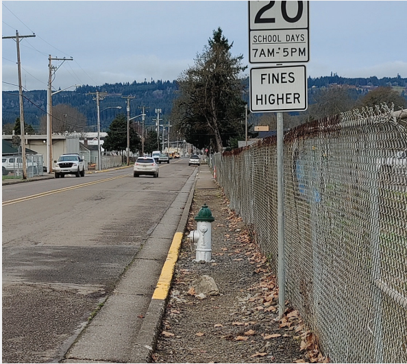
There are sidewalk gaps adjacent to Sweet Home School District property along 18th Ave (looking north).
