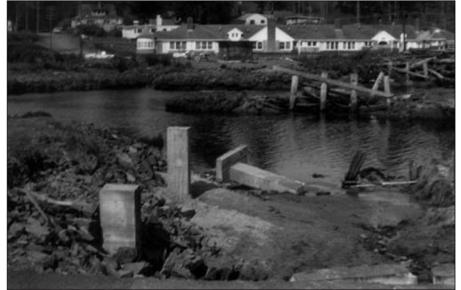
The tsunami generated by the 1964 Great Alaskan Earthquake (magnitude 9.2) caused over $250,000 dollars in damage and destroyed the Elk Creek Bridge in Cannon Beach.
