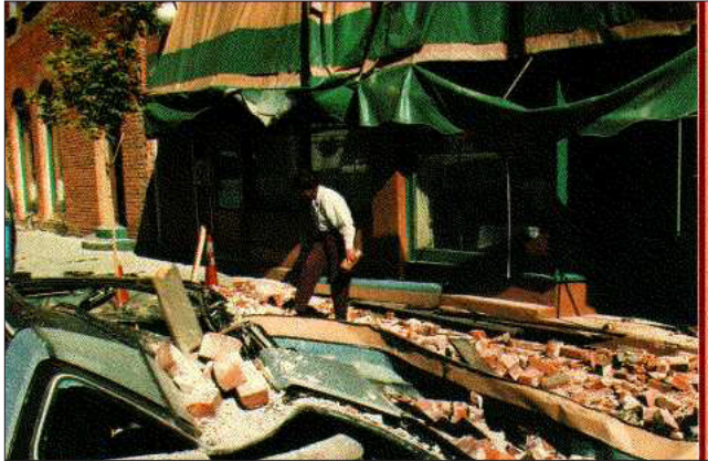
Downtown Klamath Falls after two magnitude 6.0 earthquakes in 1993. These were the largest earthquakes in history.
