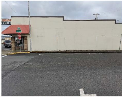
Liquor store at Thirteenth and Main
