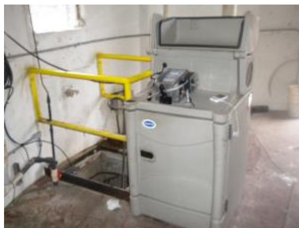
Figure 4-9. Influent flow sampler at IPS wetwell hatch
