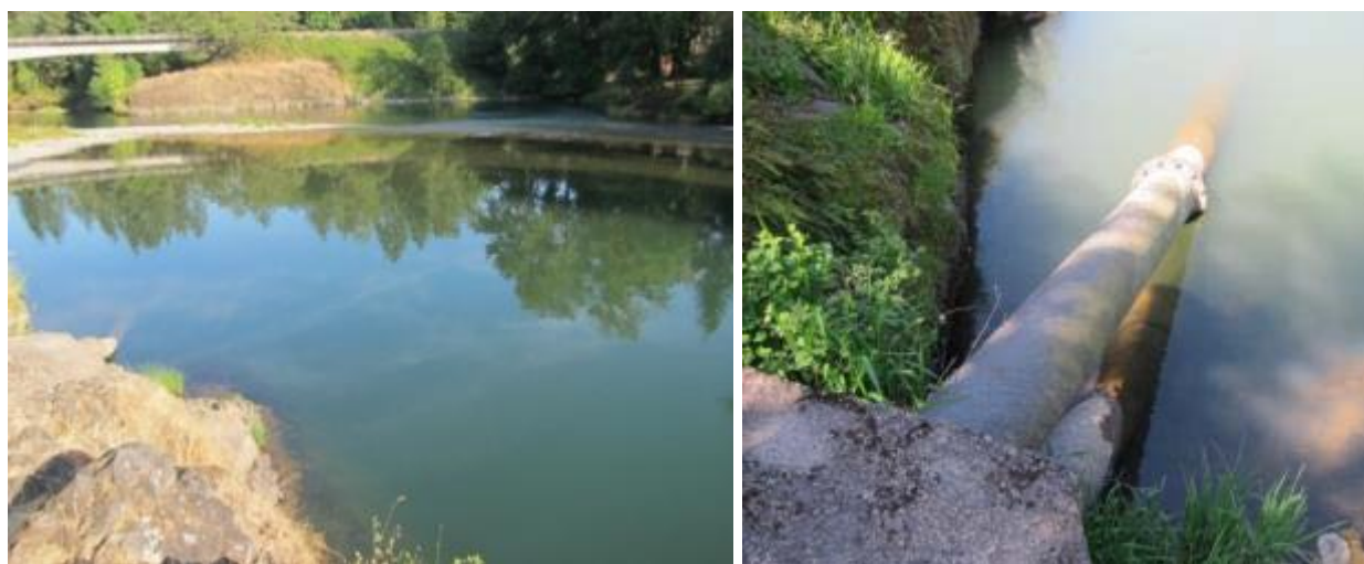
Figure 4-16. Outfall vicinity (left) and outfall pipes (right) (lower pipe abandoned)
