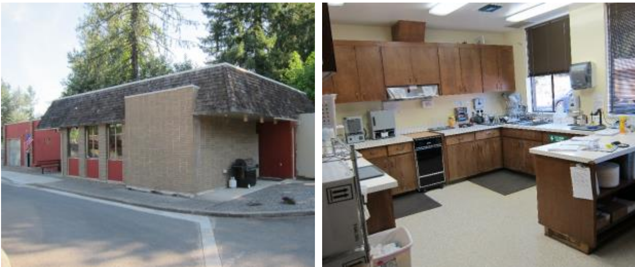
Figure 4-18. Administration building (left) and laboratory (right)
