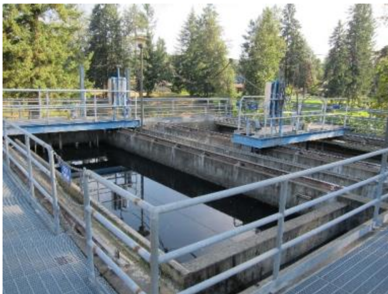
Figure 5-14. Gravity filters with sand media
