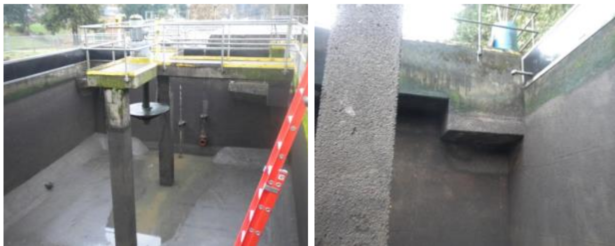
Figure 5-9. Interior of aeration basin
