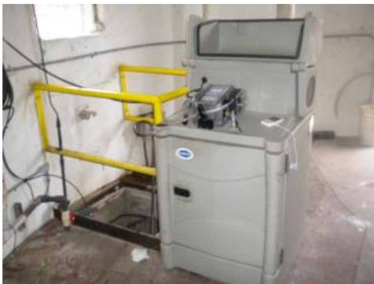
Figure 5-7. Composite sampler at IPS wetwell
