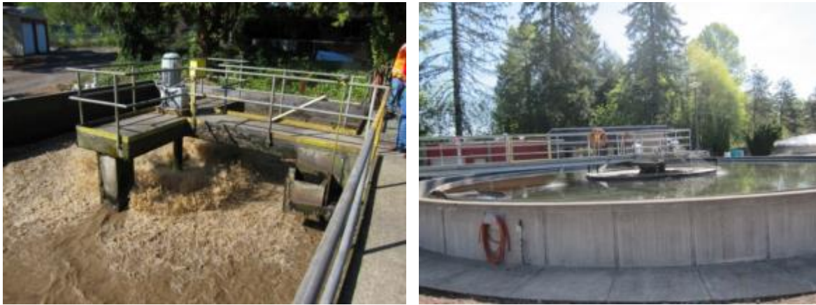
Figure 4-11. Aeration basin 1 (left) and secondary clarifier 3 (right)
