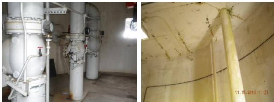
Figure 5-6. Existing IPS interior
