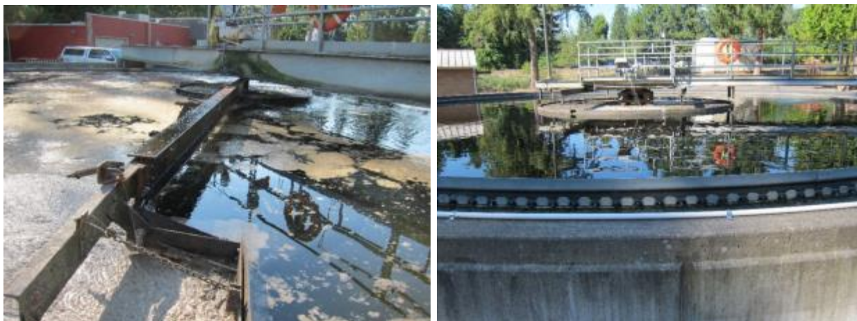
Figure 5-10. Original secondary clarifier 1 (left) and newer clarifier 3 (right)
