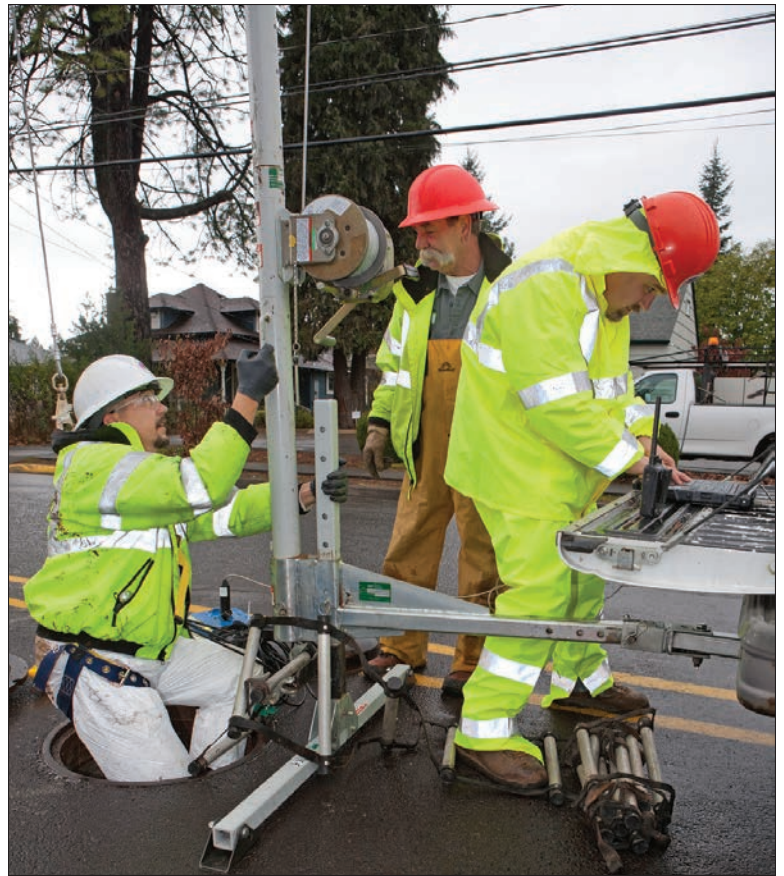
Dominic Valloni, left, is lowered into a manhole as Doug Latham and Dean LeBret adjust an ultrasonic flow device (Teledyne Isco) and calibrate area velocity.
