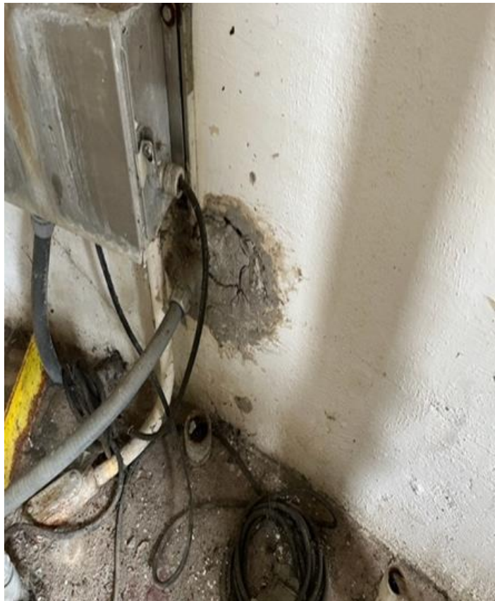
Right Holding Tank - Patch Material - Interior
