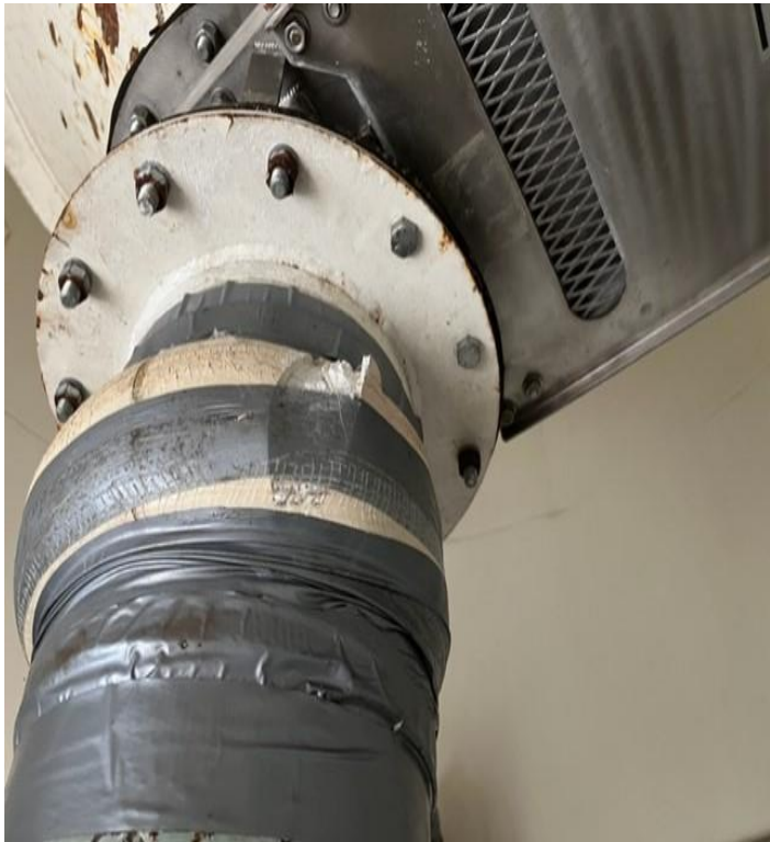
Lime Tower Insulation - Interior at funnel
