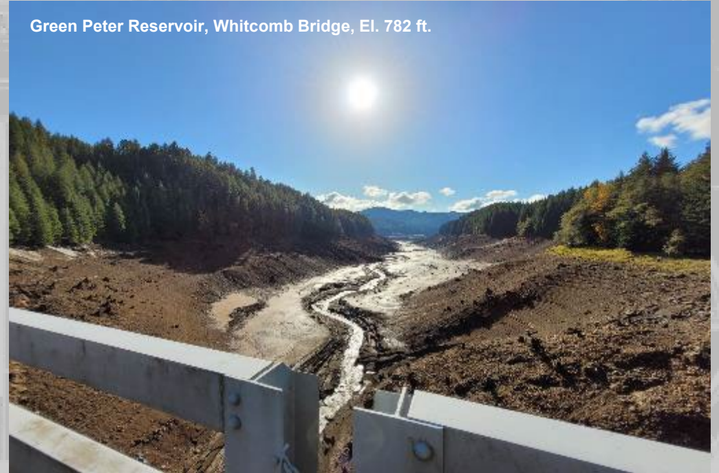
Green Peter Reservoir, at El. 782 ft.
