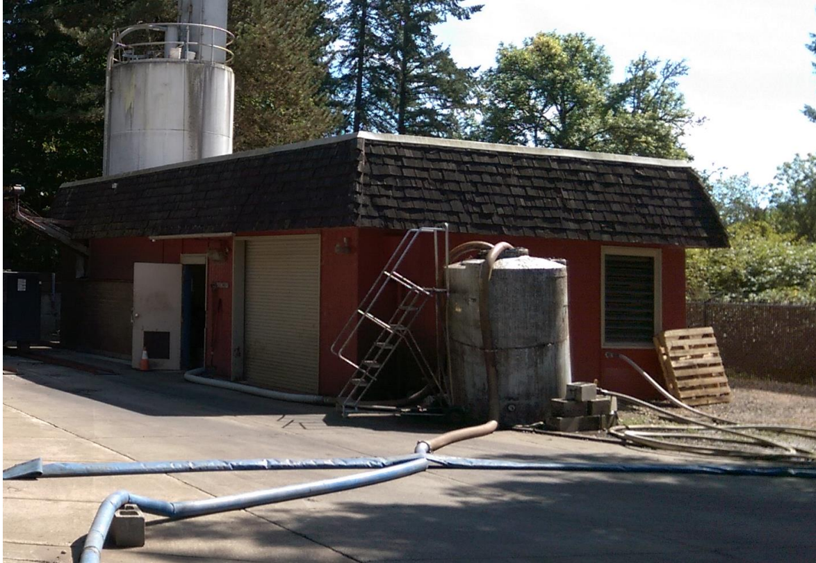
Demolish Existing Dewatering Facility
