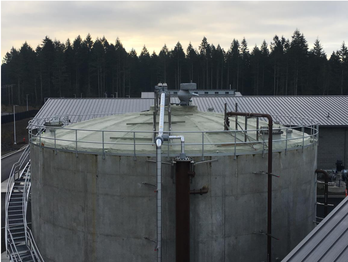
Construct new Primary Anaerobic Digester
